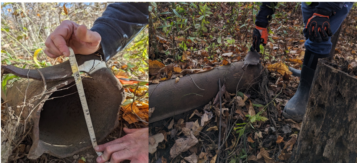
Figure A4 – Identified casing pipe at Site B.
