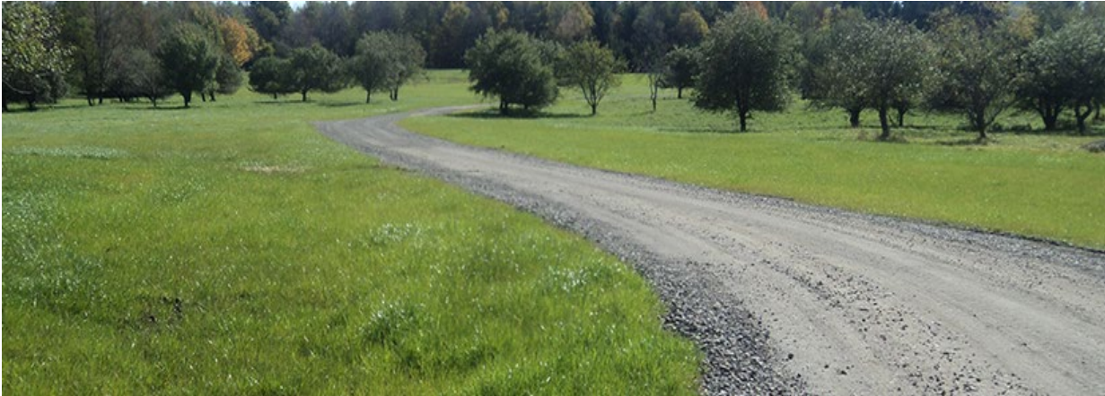
Figure 2.2-5. Representative Photo of Access Road
